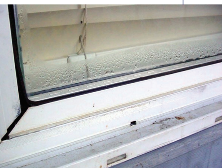
Condensation forms first on the coldest surfaces of a room, usually on glass surfaces of windows and doors.
